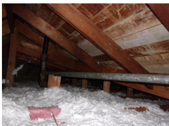
Insulation above the library
