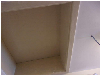
Attic Hatch to main attic
