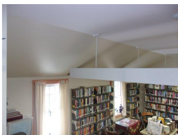
(2) Ceiling and slope Library
