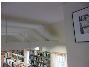
(1) Ceiling and slope Library
