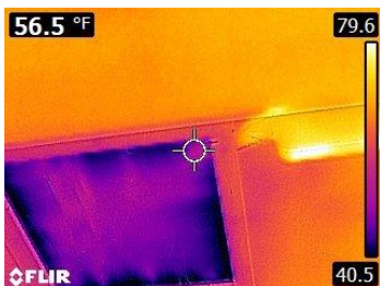
Attic Hatch - Dark area is cold
