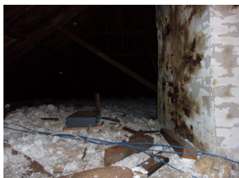
Insulation in the main attic to be removed
